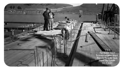
The army undertook a major construction project at Horseshoe Cove, building a submarine mine wharf to accommodate the large mineplanter ships. The new wharf, constructed with concrete and pilings, abutted the existing 1903 quartermaster supply wharf. Note Fort Bakers' open landscape in the background. (photo 1937)
