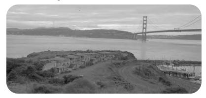
Battery George Yates, completed in 1905, is an excellent example of coastal fortification from the Endicott's period (1890 to 1905). Made of massive amounts of unreinforced concrete, this battery was constructed deep and low into the earth. Its stout construction and low-profile made it difficult for enemy gunfire to locate and attack. (photo circa 1973)
