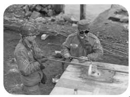
Soldiers of the 561st Port Construction Engineer Company bending rebar for a construction project. (photo circa 1960)
